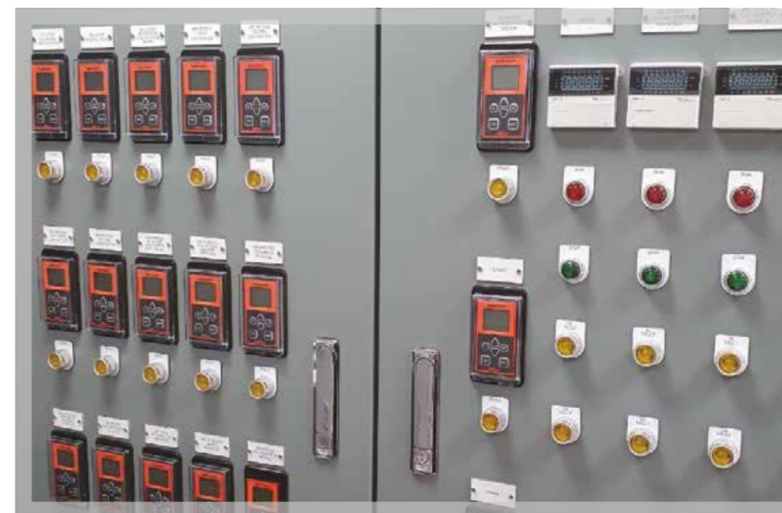
DGF-D11F (vertical type) case of ground fault relay installation switchboard
